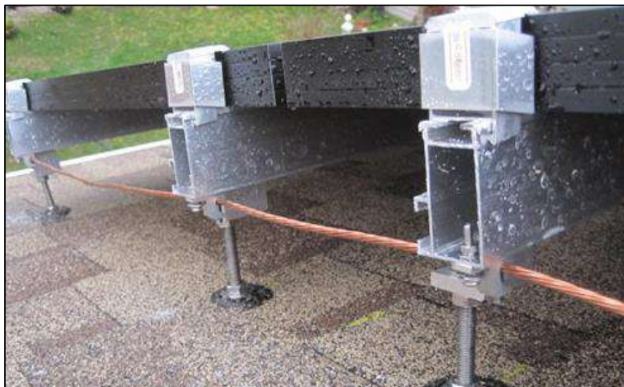
Figure 3-2: Earthing of PV Modules
