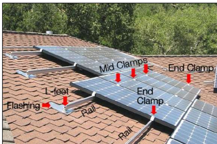
Figure 4 1: Mounting arrangement of PV modules
