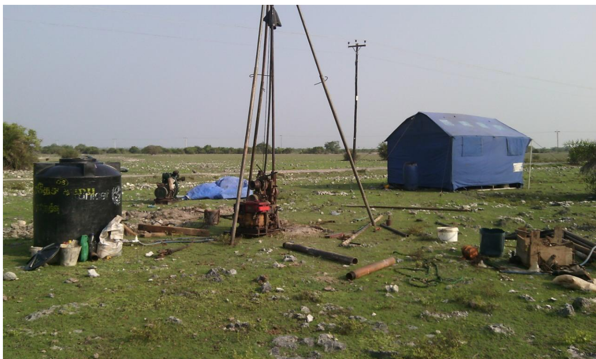
Figure 4 SPT testing and Diamond Rock Core drilling is in progress at Delft
