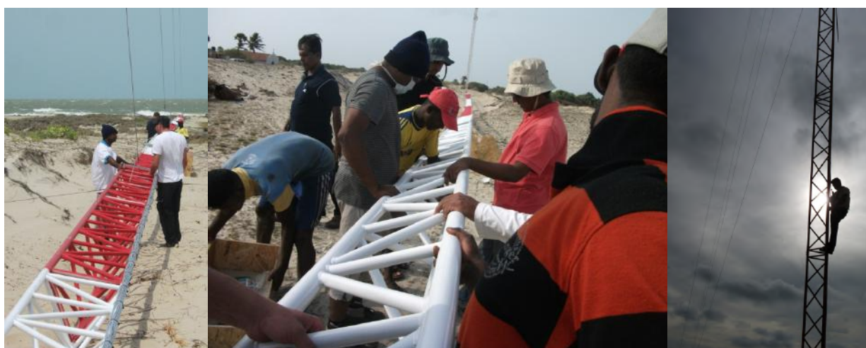
Figure 5: Installation of the 80 m wind mast in Nadukuda
