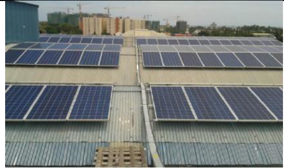
Installation of 100kWp Solar System at MJF Teas Paliyagoda
