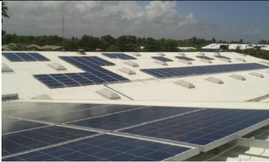
Installation of 100kWp Solar System at Brandix, Koggala
