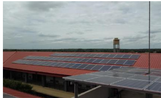
Installation of 60kWp Solar System at University of Jaffna
