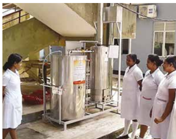
Hot Water Boilers for Karawanella Hospital by the Sustainable Biomass Energy Project
