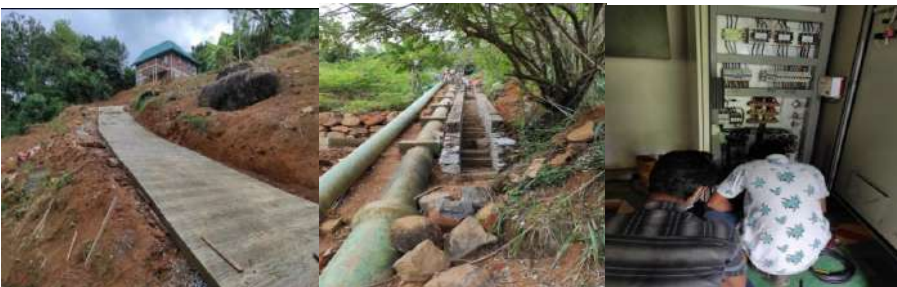
Civil construction work and lightening protection system installation
