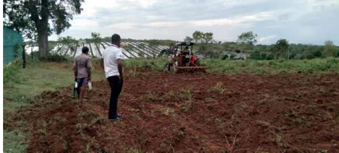
Land clearance in Hambantota Solar Park
